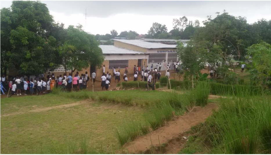
Another view of the school - Ensuring erosion control also beautifies the 'campus'
