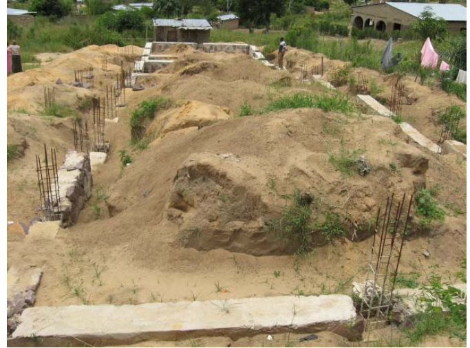
Foundation of future school
